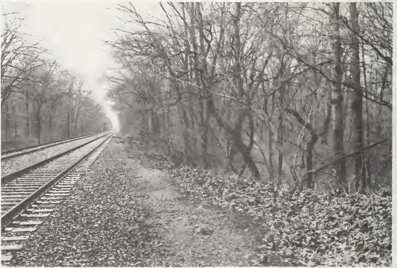
2. RR ROW - Encroaching Vegetation - Looking East
